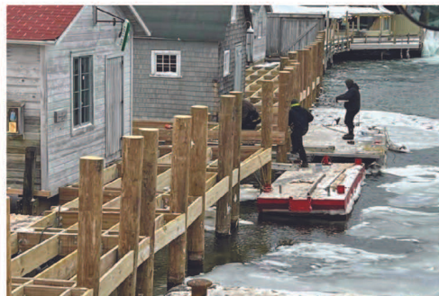
Dock framing February 2022.
