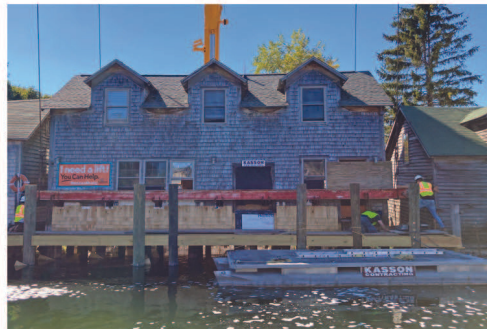
Returned to new foundation, September 2021.
