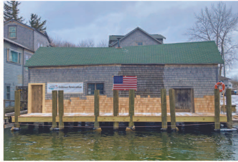
Returned to new foundation, November 2020.
