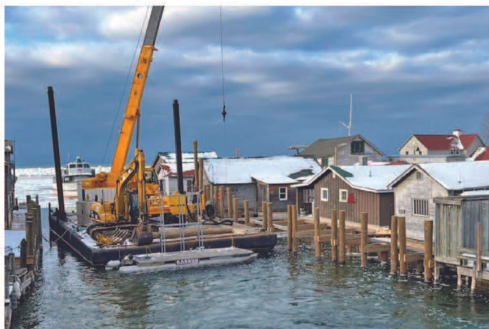
Dock piles driven January 2022.
